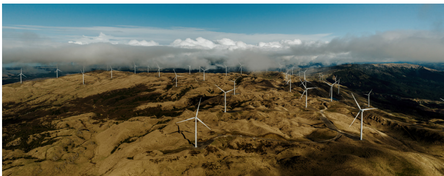
View of the Harapaki wind turbine site.
