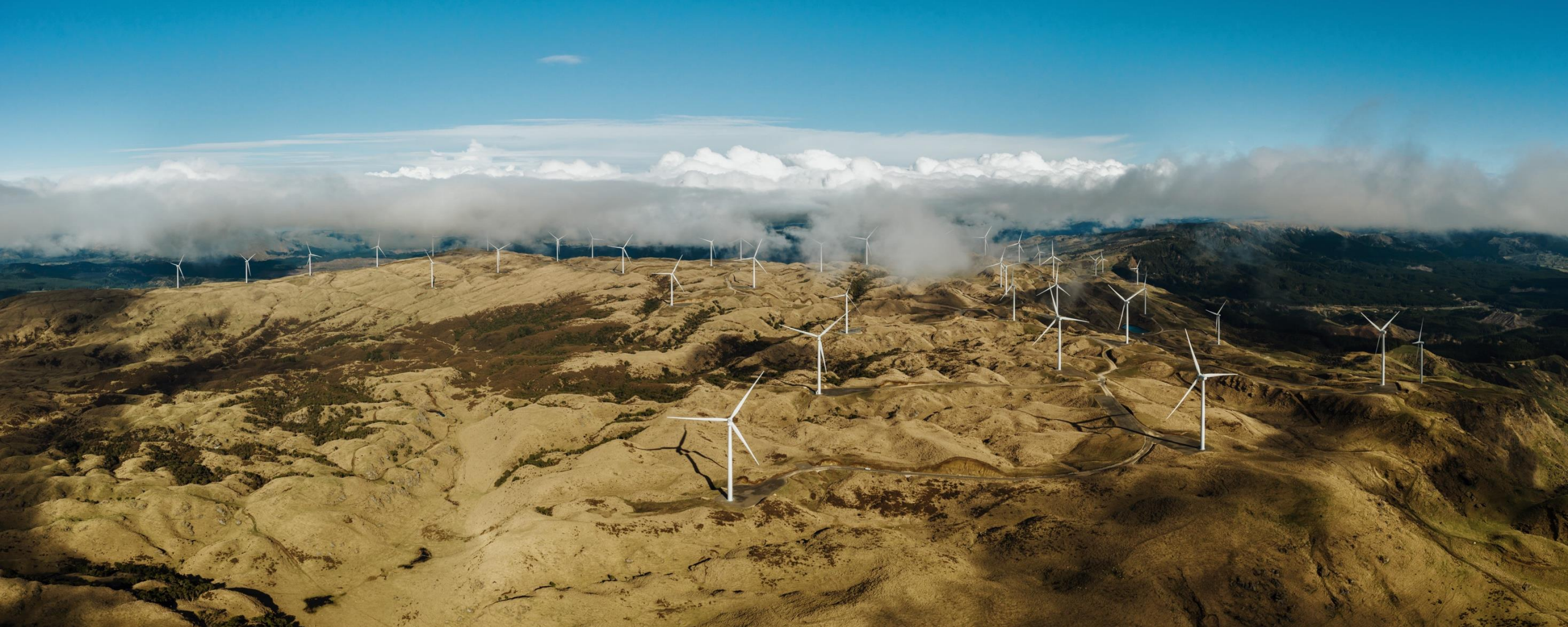
Meridian's completed Harapaki Wind Farm in Hawke's Bay
