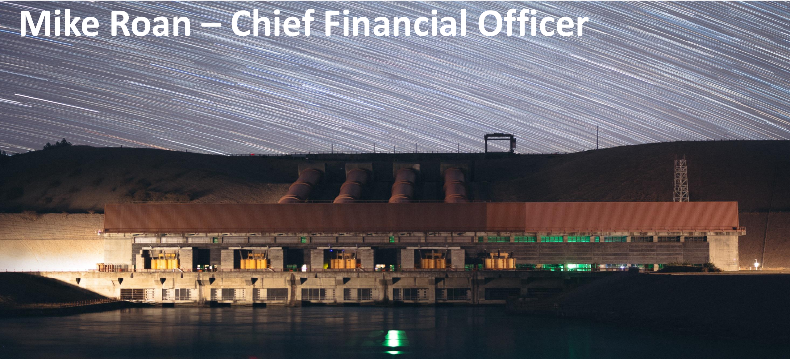
Ōhau A hydro station in the Mackenzie Basin, South Canterbury
