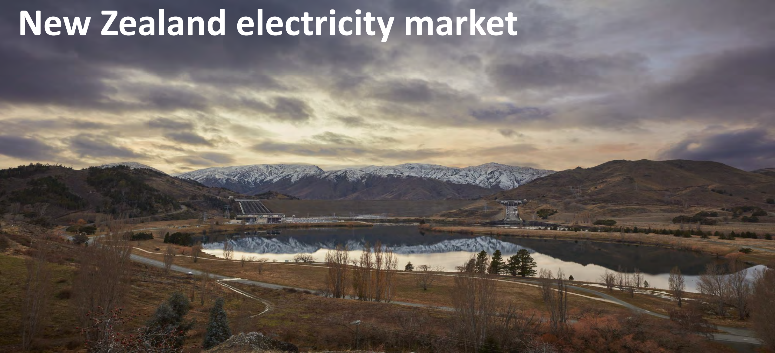
Meridian's Benmore hydro station in the Mackenzie Basin, South Canterbury
