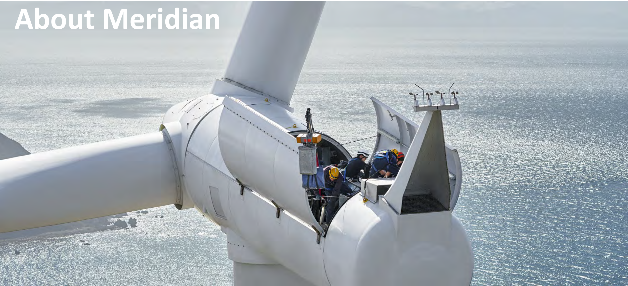
Maintenance work at Meridian's West Wind Farm near Wellington
