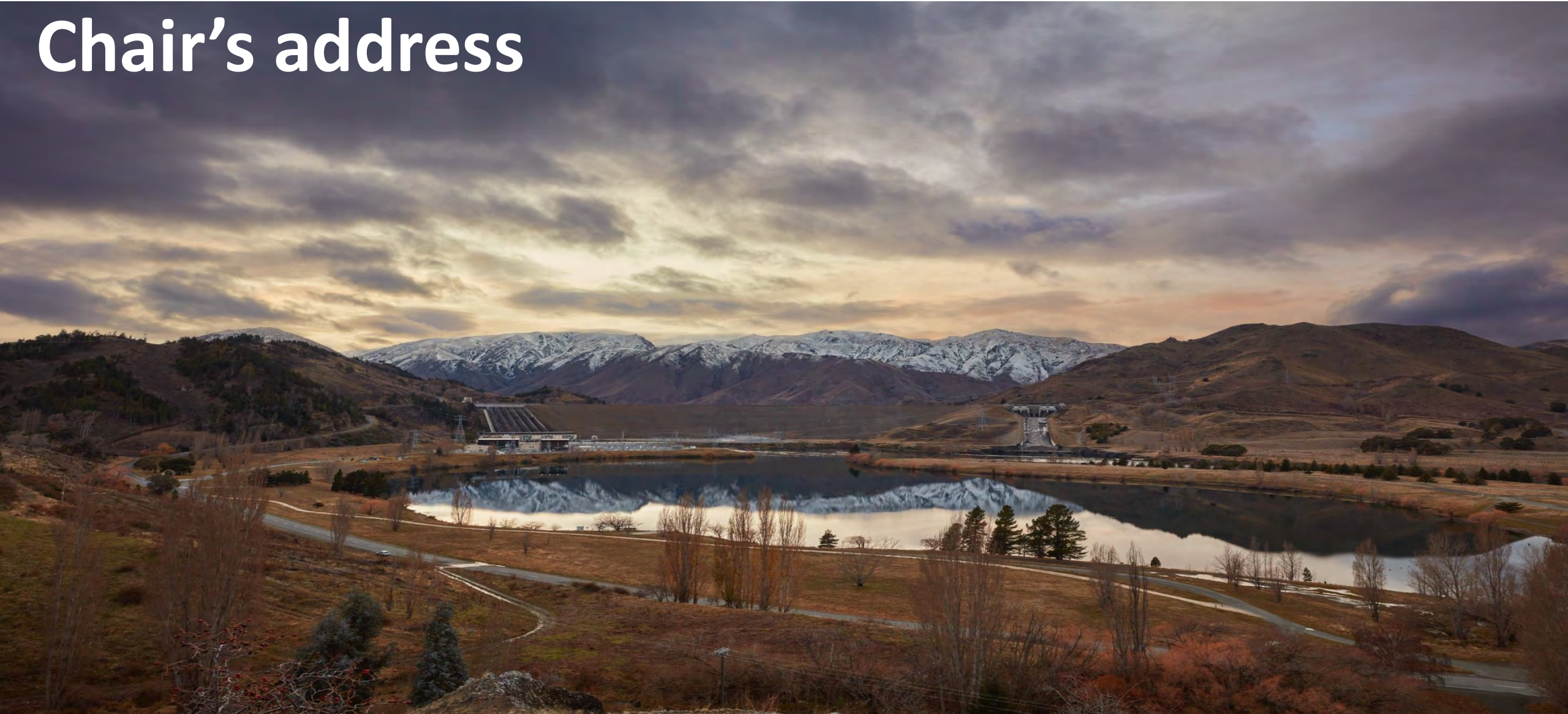
Benmore hydro station in the Mackenzie Basin, South Canterbury
