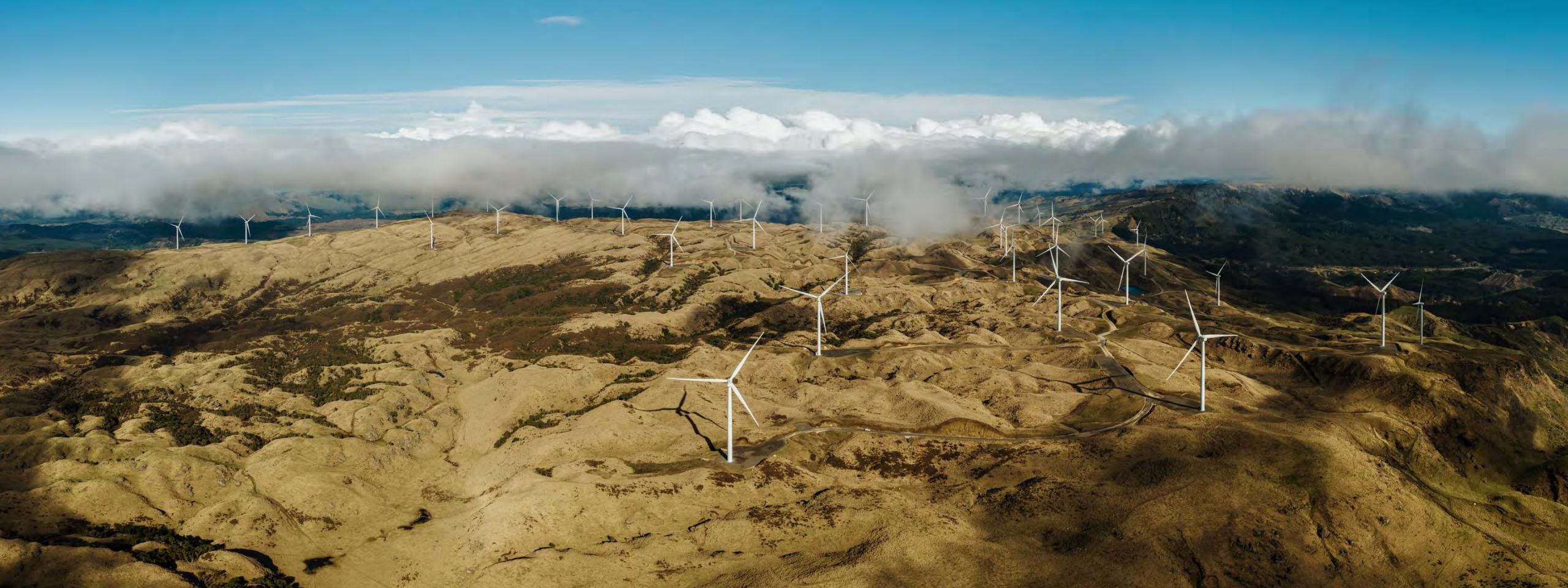
Meridian's completed Harapaki Wind Farm in Hawke's Bay
