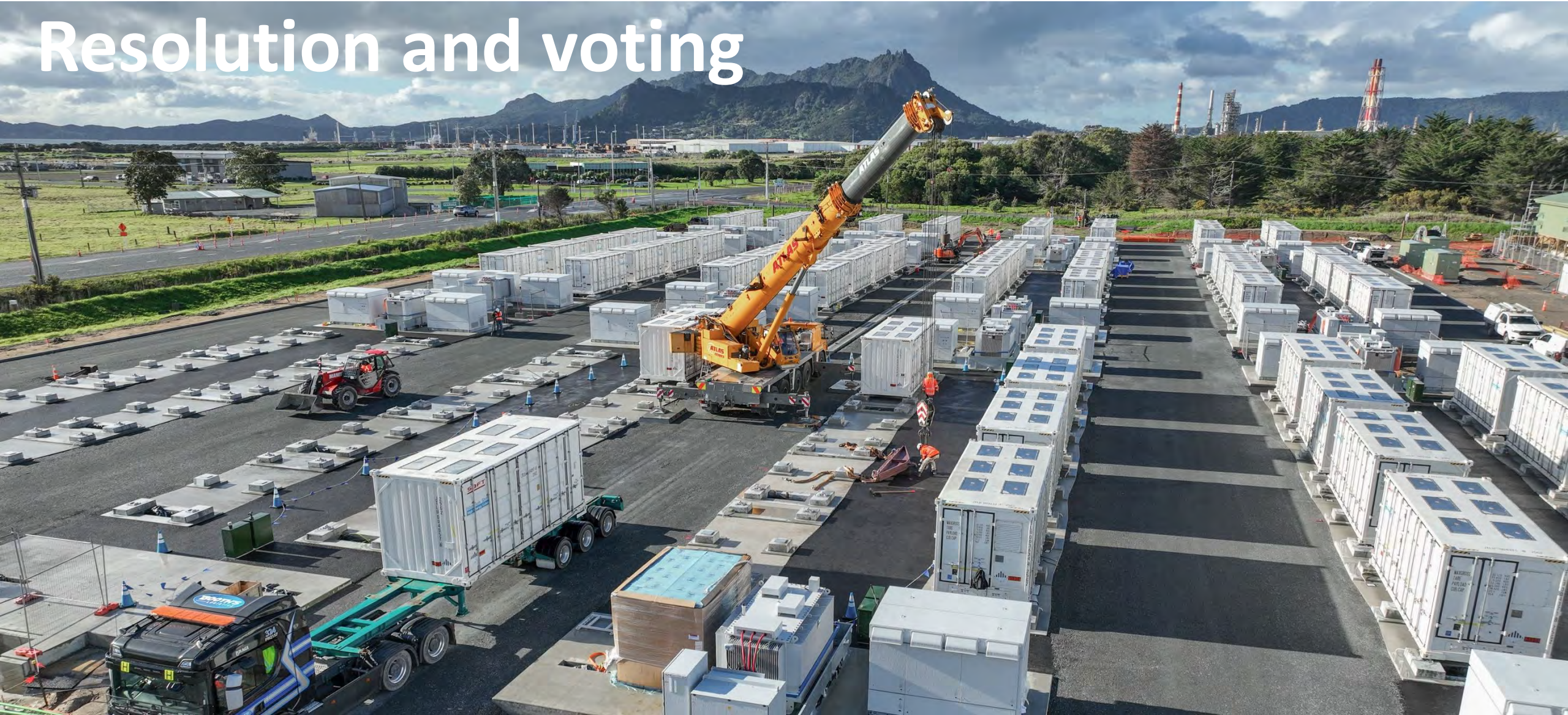
Container installation at Meridian's Ruakākā Battery Energy Storage system near Whangārei
