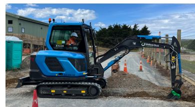
United Civil's e-digger at work on site
