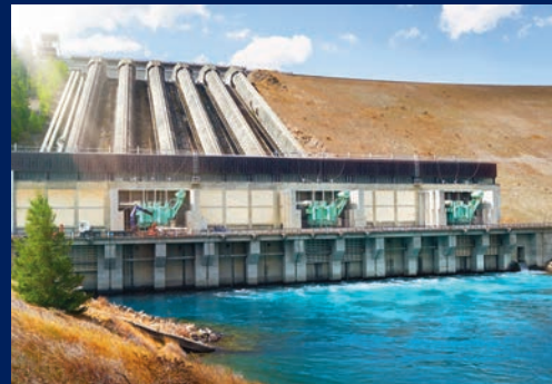
Benmore Hydro Station
